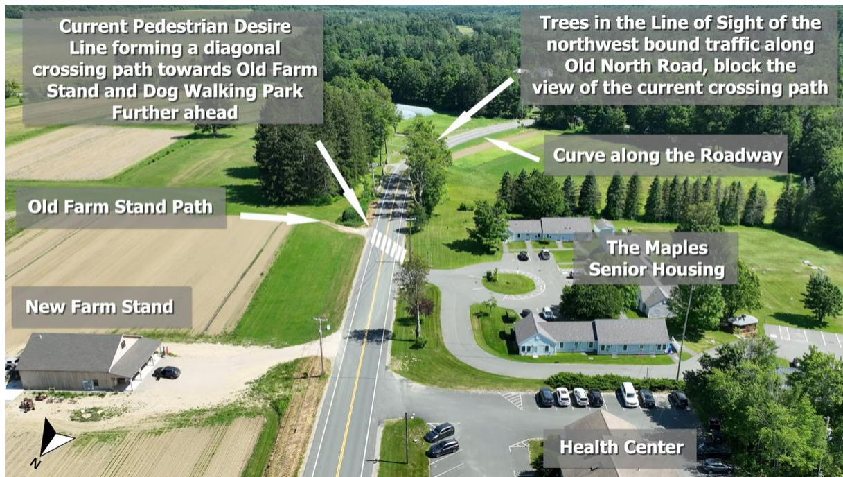
Figure 2: Drone Image of the Study Area (facing East/Southeast)
