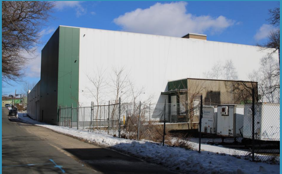
83-95 Warwick Street, viewed from the southwest
