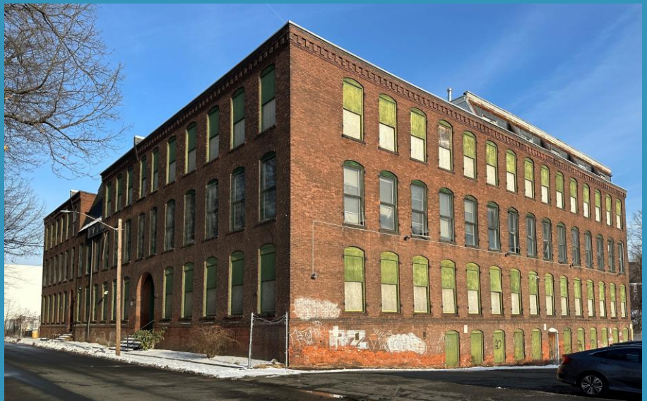
The building at 45 Warwick Street, viewed from the southwest
