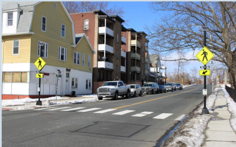
New sidewalks and crosswalk on Liberty Street at the corner of Tracy Street
