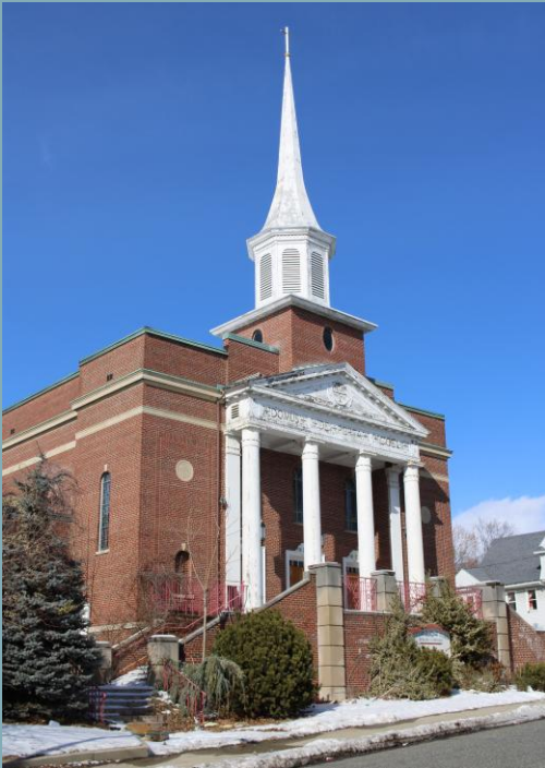
The former church at the corner of Franklin & Underwood Streets
