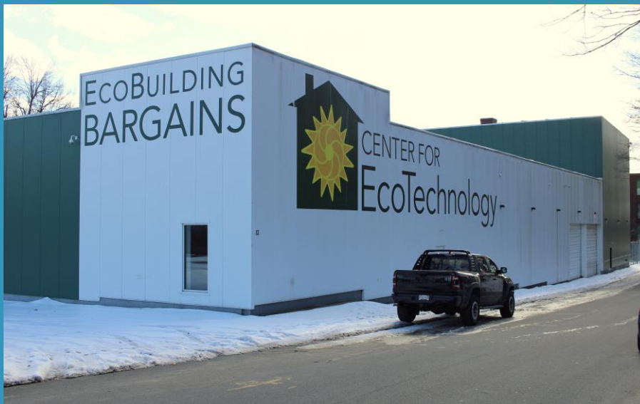
The building at 83-95 Warwick Street, viewed from the north
