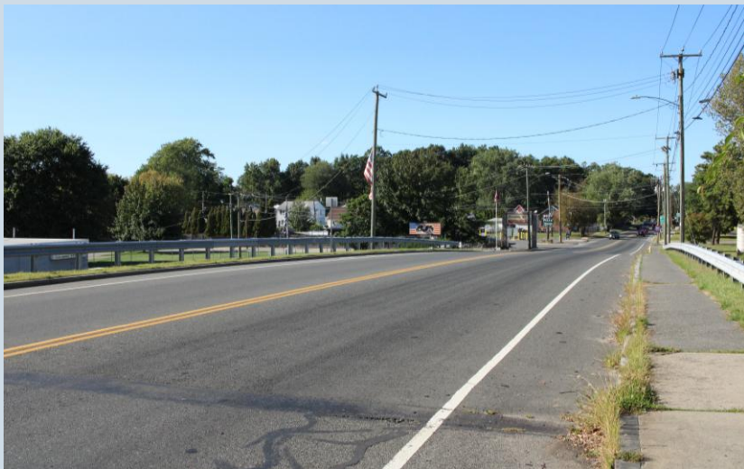
Pasco Road (US Route 20) facing north toward Page Boulevard
