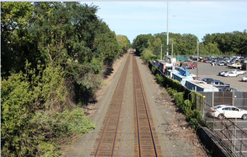
The CSX mainline forms the southern boundary of the Indian Orchard neighborhood. View looking east from Pasco Road bridge.
