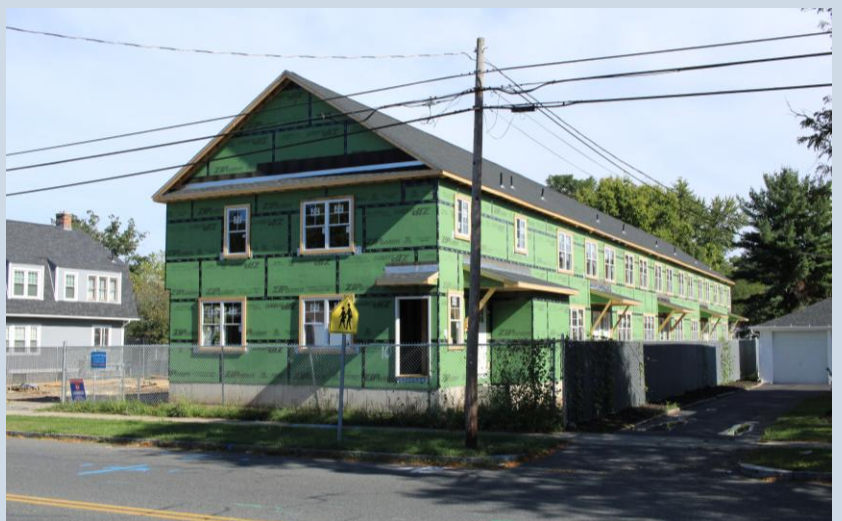
New housing under construction on Parker Street in Indian Orchard
