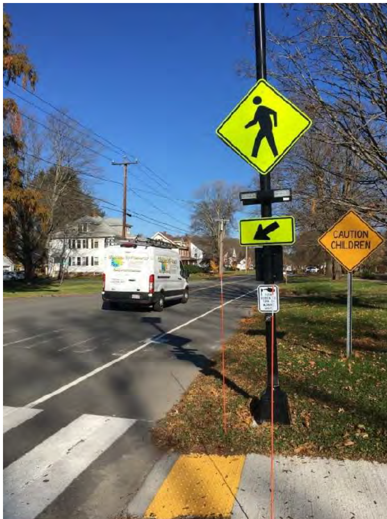
Hatfield DPW installed Rectangular Rapid Flashing Beacons pedestrian actuated signals on the Main Street intersection with North Street in 2023 as an effective safety initiative.
