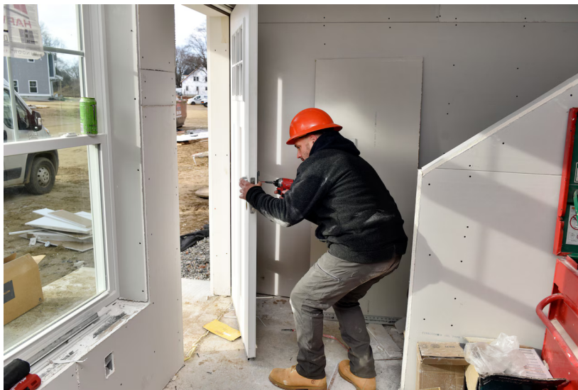
Carpenter Paul Pennell of Holyoke installs door hardware on a unit at Rosewood Way, Wayfinder's new affordable and market rate housing development in Agawam. (Don Treeger / The Republican) 12/14/2023
