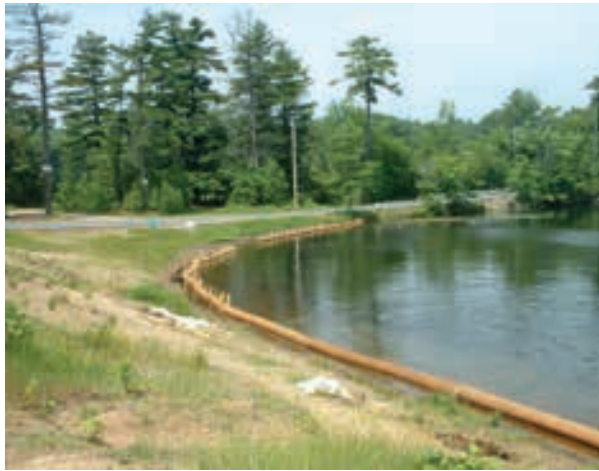
Pequot Pond restoration project, Southampton
