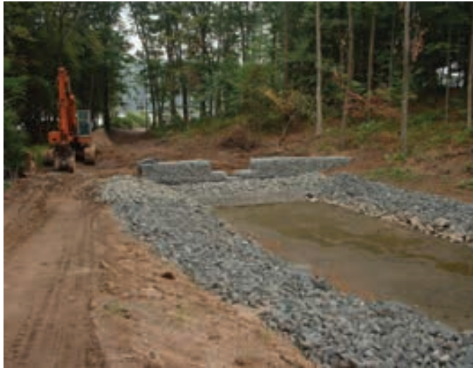
Congamond Lakes Restoration Project, Southwick
