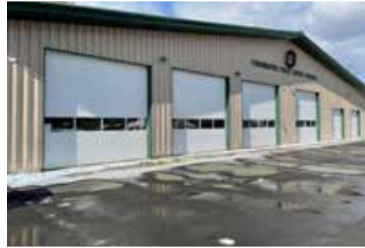
Figure 33 Cummington Fire Front view
