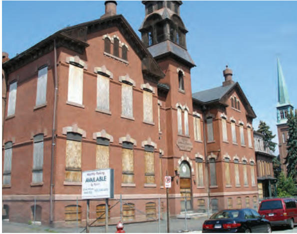
Former Holyoke Catholic High School
