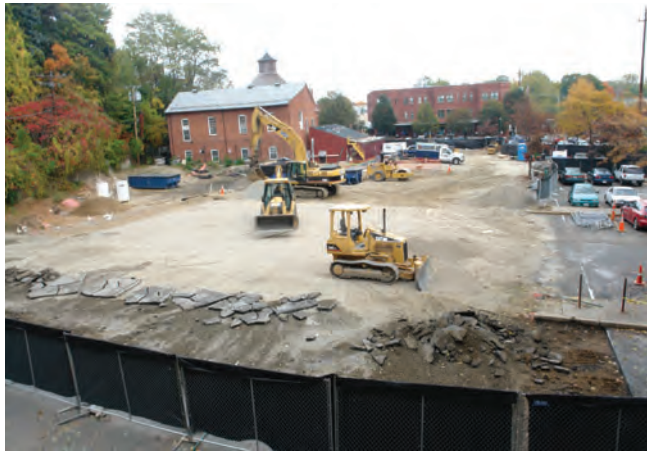
Roundhouse Parking Lot project, Northampton
