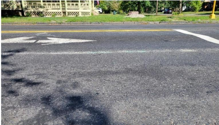
2. The St. James Avenue southbound approach does not have crosswalk markings connecting the sidewalks on both sides of the street. The current Stop line at this approach is located behind the ADA ramps for sidewalks to the north of the intersection. It is possible that there was a crosswalk painted at this location in the past which was not repainted. It is recommended that the City install a crosswalk at this location to provide connectivity for the sidewalks along both sides of the pavement.
