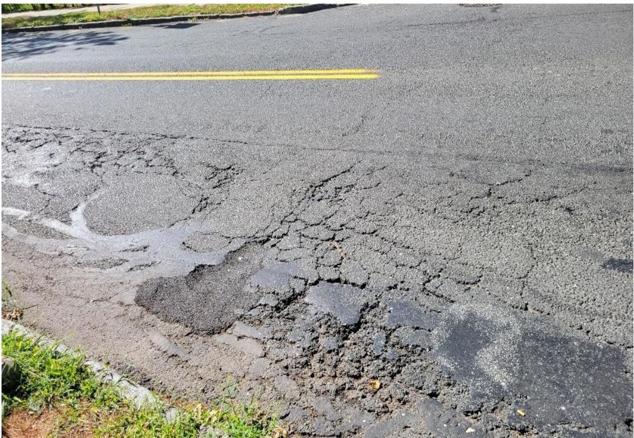
*Figure 13: St. James Avenue Faded Pavement Markings and Pavement Rutting*
