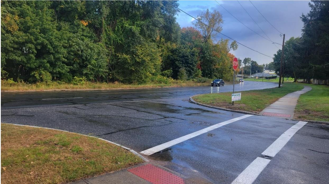
Roosevelt Avenue is a four-lane undivided highway classified as urban minor arterial which is aligned in the northeast-southwest directions in the vicinity of the study area. Streetlights are installed along the west side of Roosevelt Avenue in the vicinity of the intersection. A speed limit sign restricting the speed to 35 mph for vehicles travelling southbound along Roosevelt Avenue is located north of the intersection.
