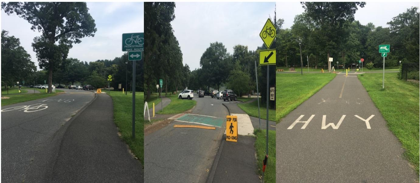
**Remarks:** This crossing is located along a one way internal road inside Look Park. The pavement markings are faded at several locations along the roadway.
