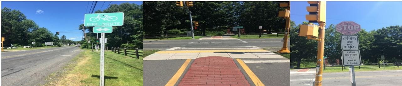
**Remarks:** The crossing is located on a high traffic volume corridor. There is a parking lot on Damon Road in the vicinity of the crossing. The crossing has a push button activated signal which allocates approximately 13 seconds of crossing time. The pavement markings and crosswalk markings need to be repainted at this crossing.
