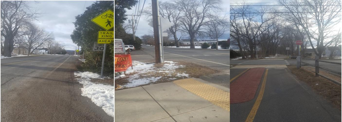
**Remarks:** The existing pavement markings have faded and the advance warning sign for East Street south bound approach is partially covered by vegetation. The sight distance to the north for the eastbound approach of the shared use path is limited because of the road geometry, existing vegetation and utility poles. The advance warning sign for the shared use path crossing along the southbound approach of East Street is partially covered by vegetation.
