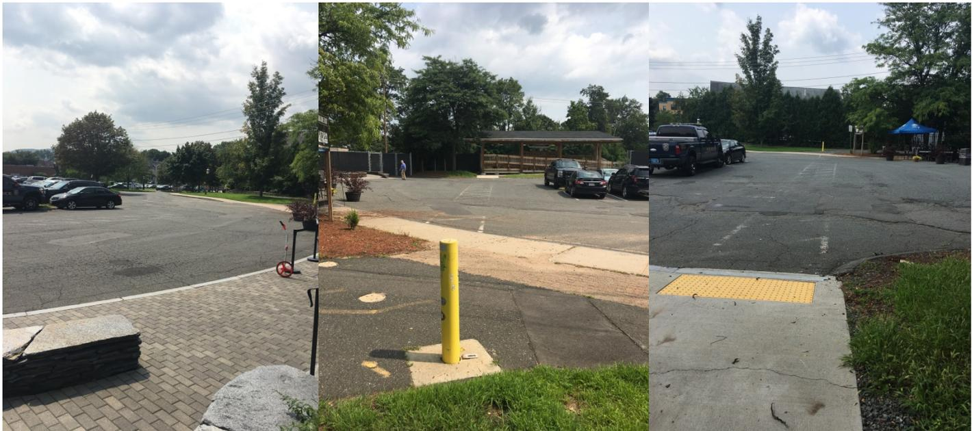
**Remarks:** This crossing is located within the Northampton Union Station parking lot. The crosswalk markings are faded at several locations. It is recommended this crosswalk be repainted.
