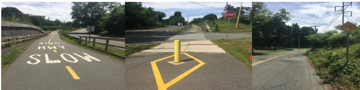
**Remarks:** The crossing is located at the three-way intersection of Lovefield Street and O’Neil Street in a residential area with a low volume of traffic. The geometry of the roadway creates sight distance issues for shared use path and roadway users.
