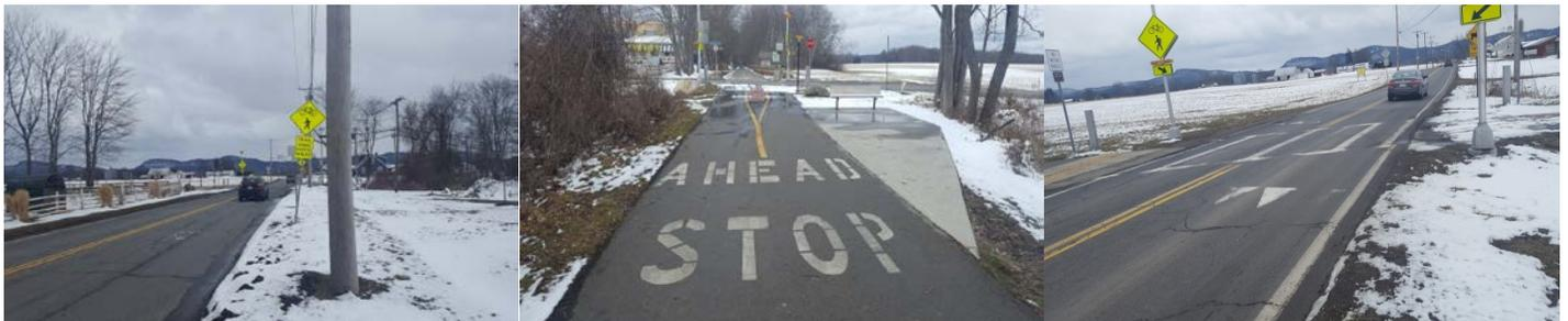
**Remarks:** Advance pavement markings along both directions of South Maple Street have completely faded. Shark Teeth Yield lines and cross walk markings at the intersection have also faded. This location has retail development in the immediate vicinity; however there are no sidewalks to connect the intersection with the retail establishments on both sides of South Maple Street.
