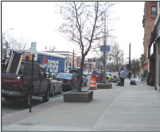
A view on North Street in Pittsfield before the City undertook the street improvement project. Here, stormwater is conveyed along street curbs to nearby catch basins (and then piped to the nearest waterway).
