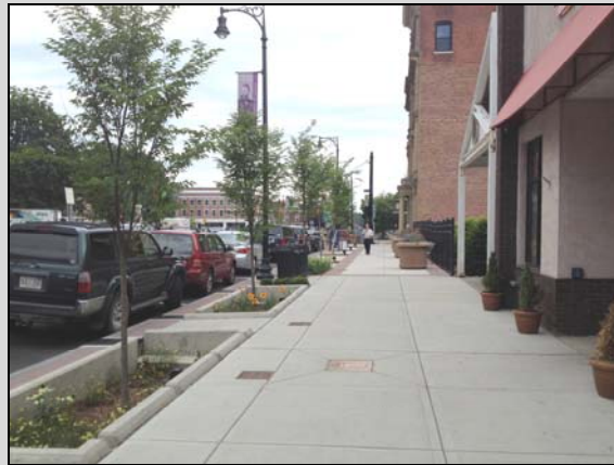
The same view on North Street showing how the new bioretention planters that receive stormwater from the street support an improved experience for pedestrians.
