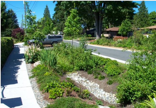
Seattle Public Utility Natural Drainage Project in the Piper's Creek watershed showing a bioretention area.
