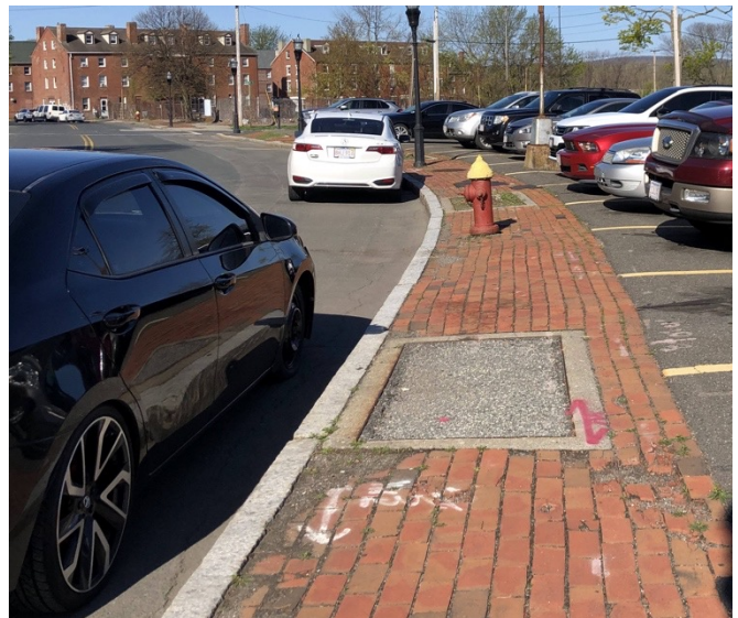
Sidewalk in front of Market Square Plaza Source: Ken Comia
