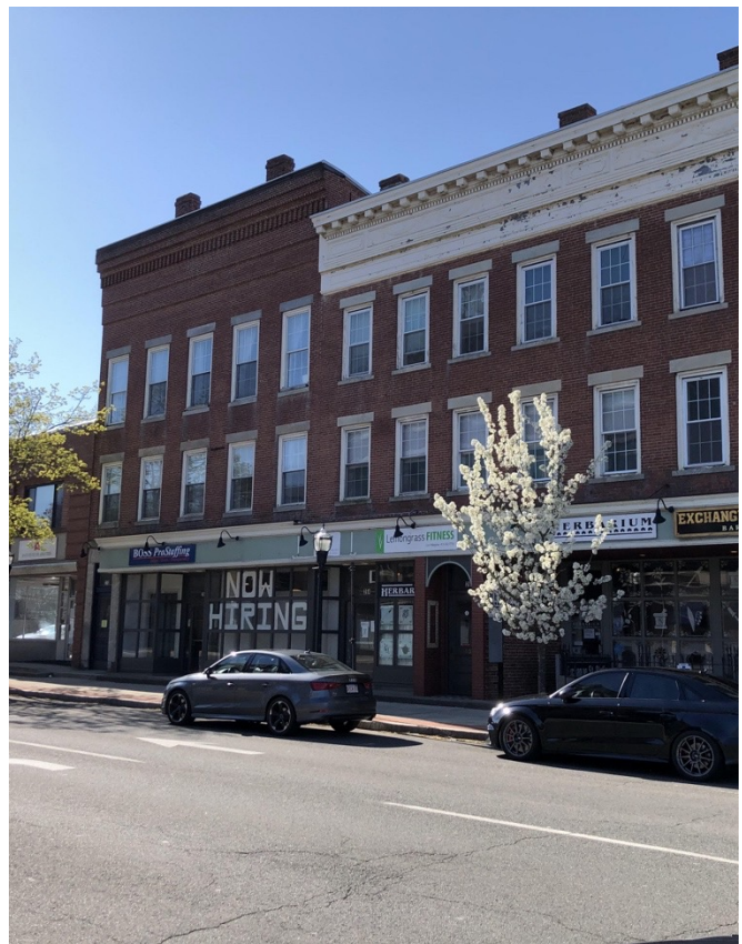
Storefronts along Exchange Street Source: Ken Comia
