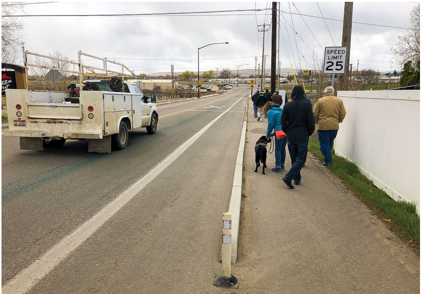
Extruded curb treatments, like these in Kuna, Idaho, are used in Emmett and other rural areas to create safe pedestrian walkways without the full cost of sidewalks. Photo by Don Kostelec.
