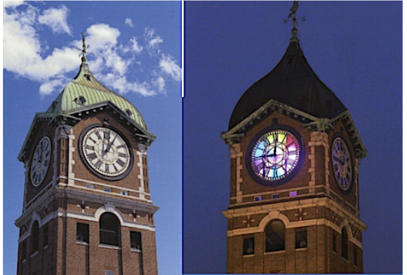
Lighting was used to emphasize significant architectural features and to enliven the downtown experience. .
