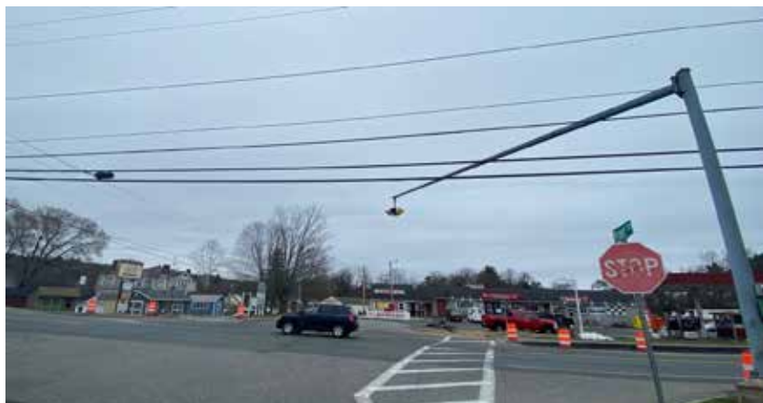
Intersection of Rte 202 and Stadler Street
