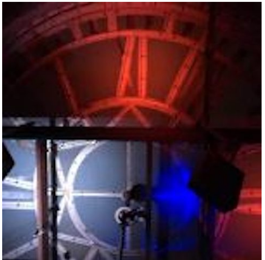
Internal view of Ayer Mill Clock Tower lighting..
