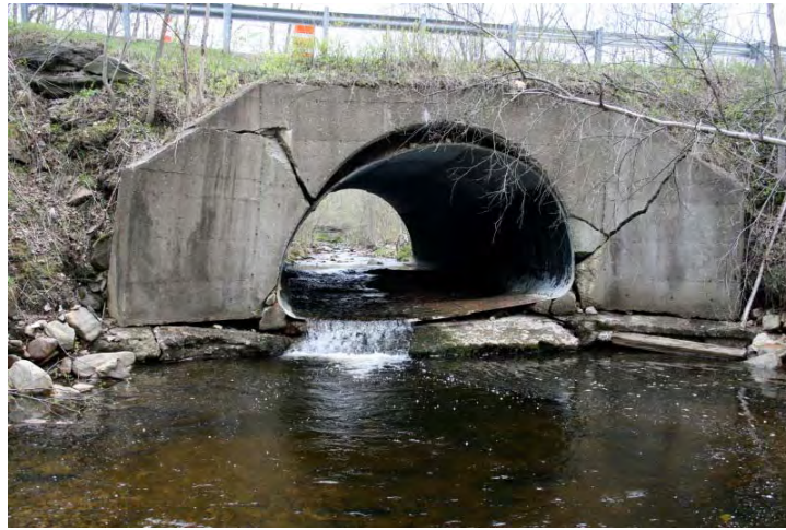
McNearney Road crossing of Shaker Brook, Becket, before. (Credit: Carrie Banks)
