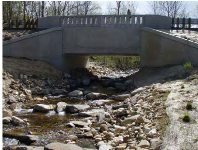
McNearney Road crossing of Shaker Brook, Becket, after. (Credit: Carrie Banks)
