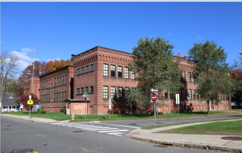
The former Brightwood Elementary School on Plainfield Street, which will be converted into affordable housing
